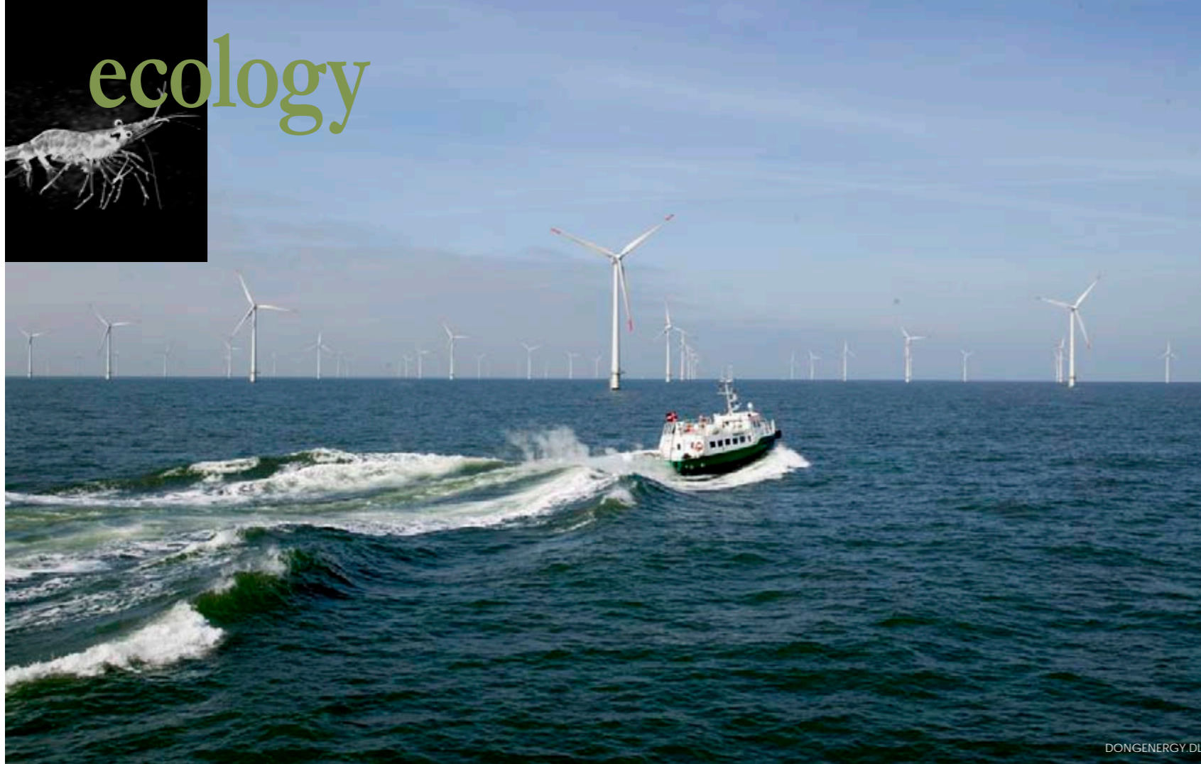
At Horns Rev, the Danish Energy company Elsam (now DONG Energy) built the first offshore wind farm in the North Sea. A total of 80 Vestas V80-2.0 MW units, capable of producing 160 MW, were installed
