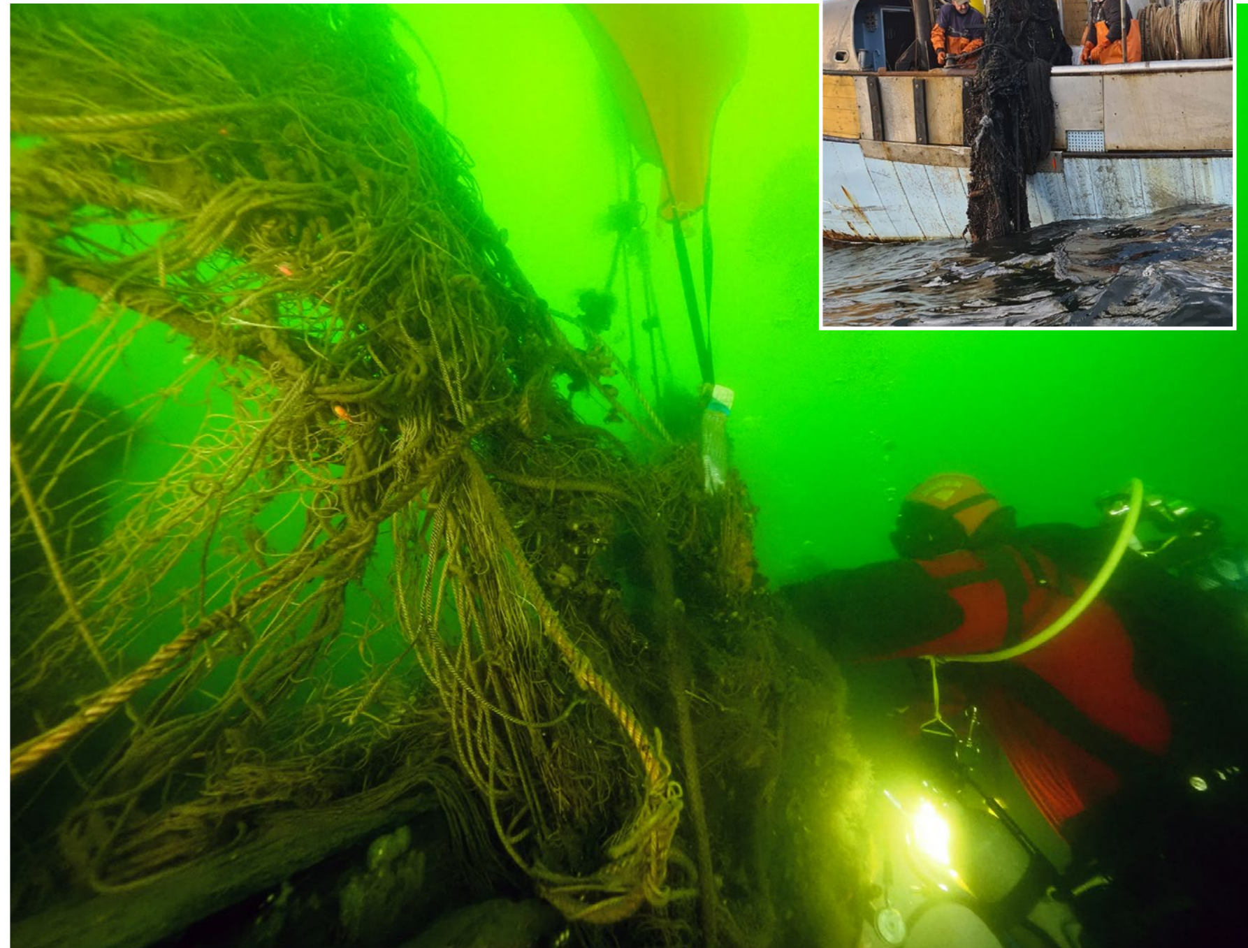
Diver attaches lift bags to nets to lift them off the Flying Dutchman near Rügen (above)
