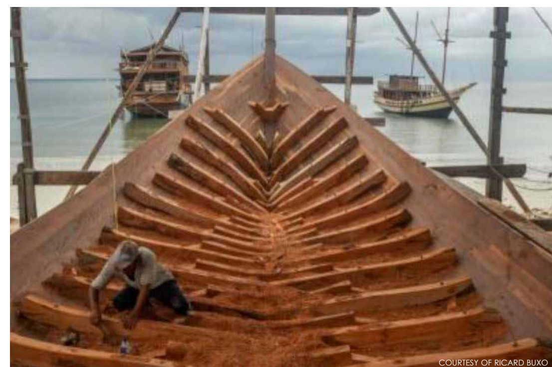
Pinisi boat building at Tanah Beru in Sulawesi (left, above and right)
