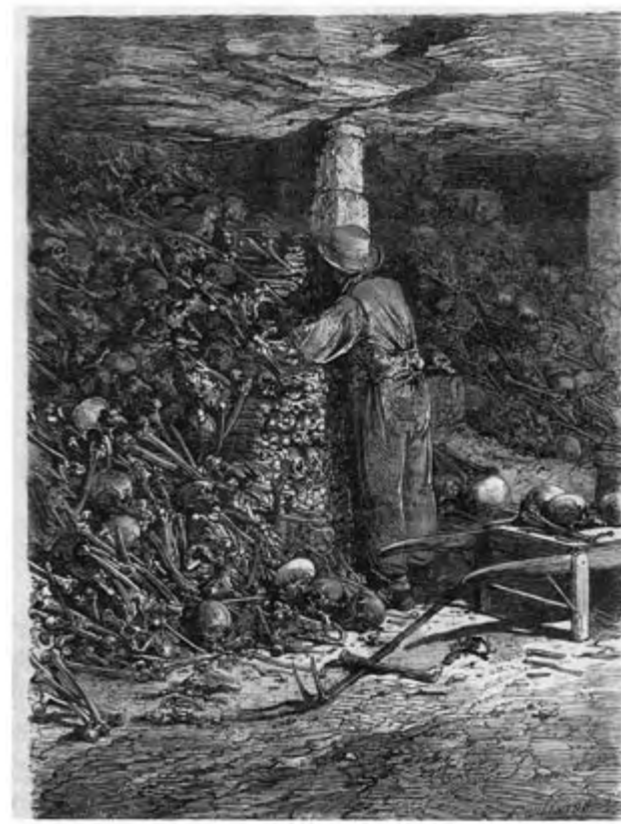
Construction of the ossuary. Litograph
