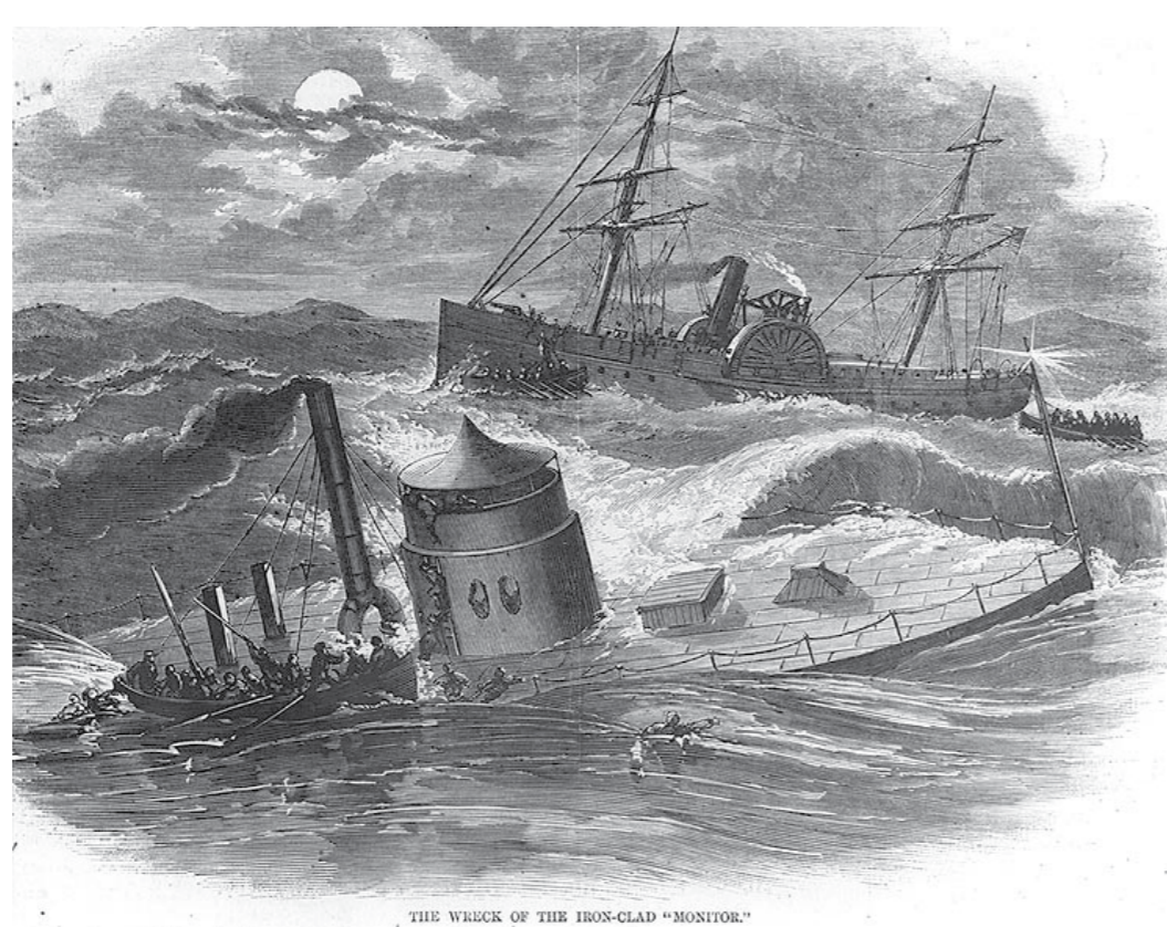
THE WRECK OF THE IRON-CLAD "MONITOR."
