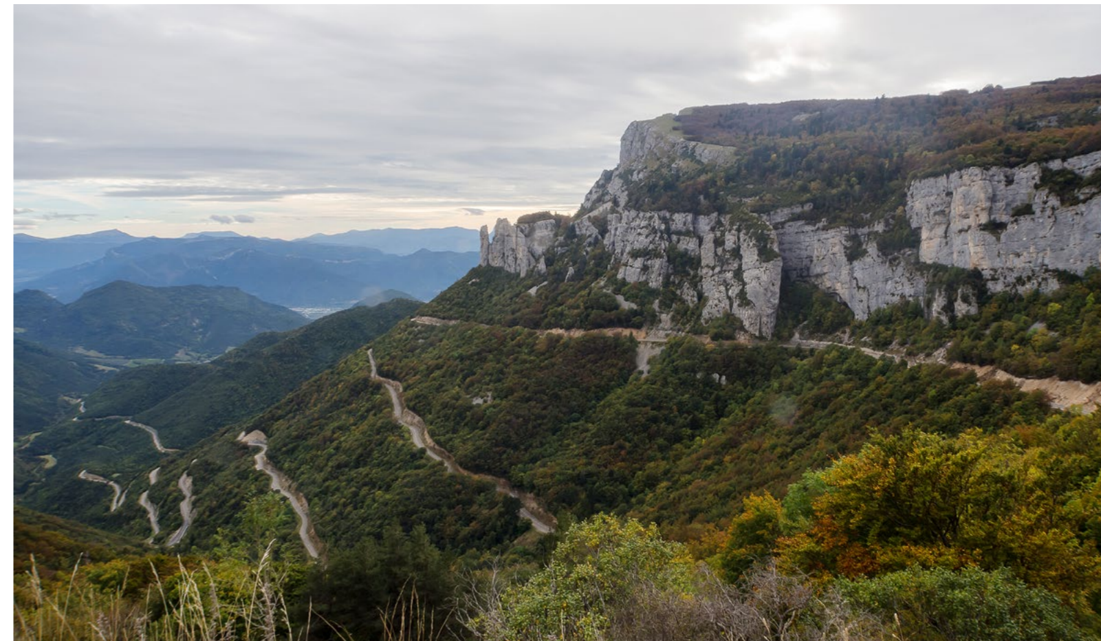
The winding, serpentine road from the town of Die ascends the high plateaus of the Vercors
