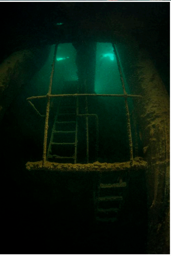
Pump house of Amatsu Maru
